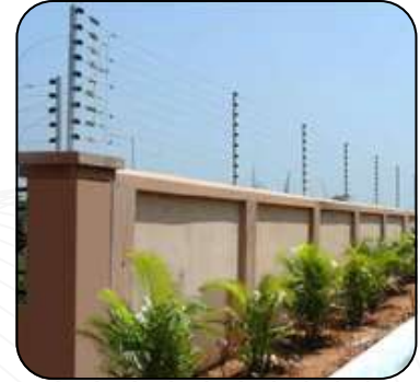
Solar Fencing 9 / 6 lines
